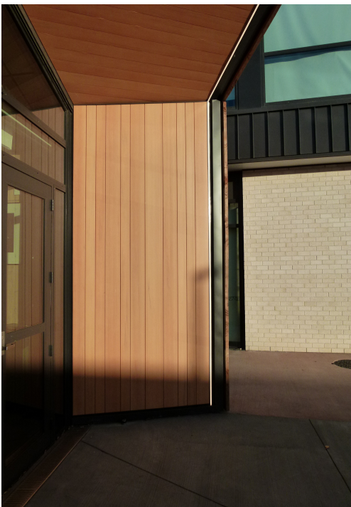
Correctly Mixed batches and boxes, achieving a natural variance & good finish
