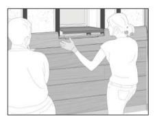
Install the trimmed plank, which now matches the window and sill. Take extra care not to break the plank where the edges have been cut out.
