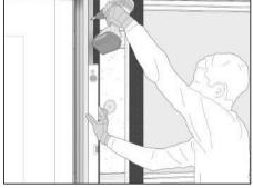
Ensure vertical profiles are installed straight and plumb
