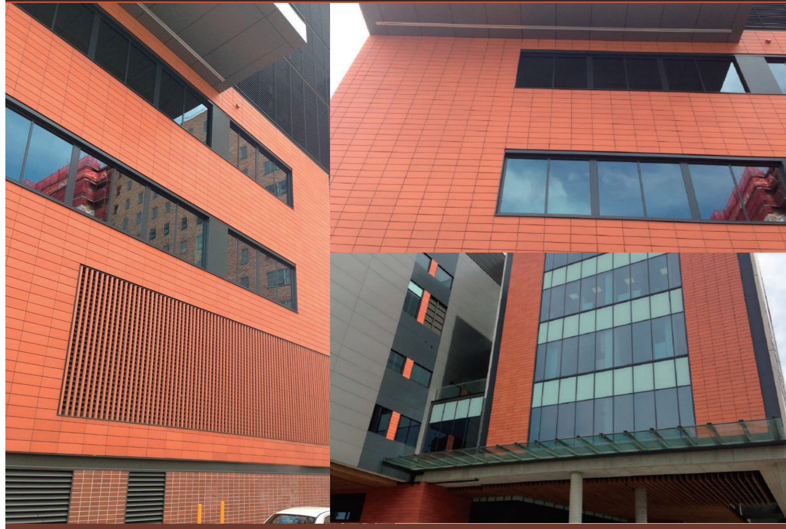
RPA Hospital, Pecknohaztel, Sydney, Australia
