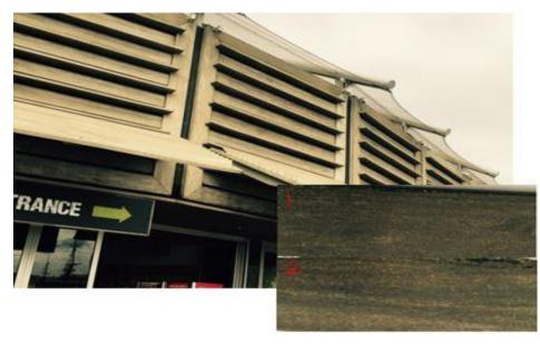
**Sample 1** - The Image of the surface after 10 years of exposure facing North/West (image taken 26 September 2016) **Sample 2** - Shows an image of the of the surface "as fresh"
