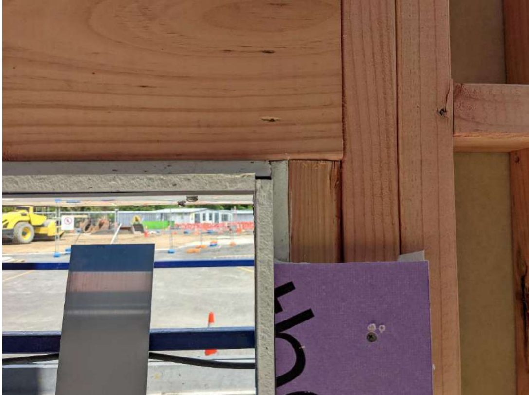
Photo 6: Combustion chamber opening – internal junction
