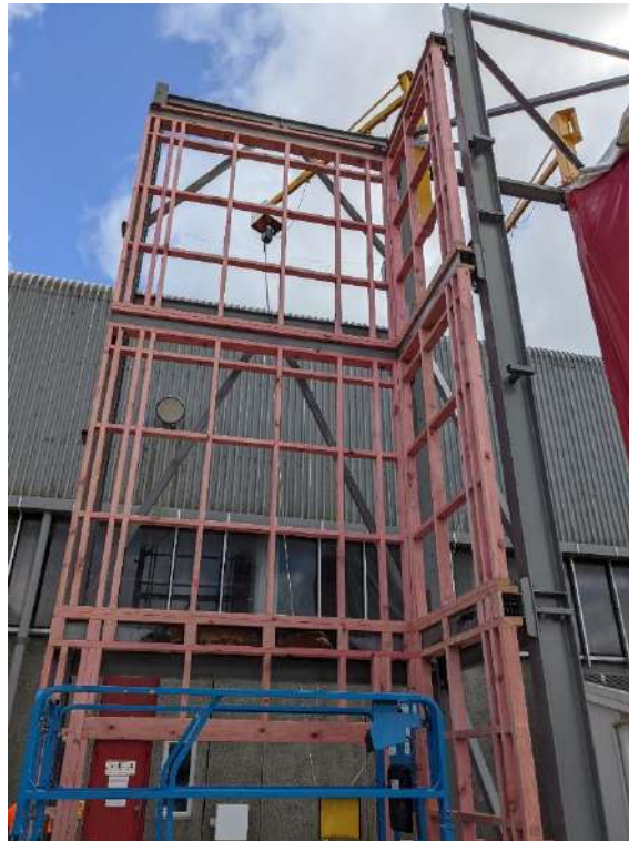
Photo 3: Structural wall frame
