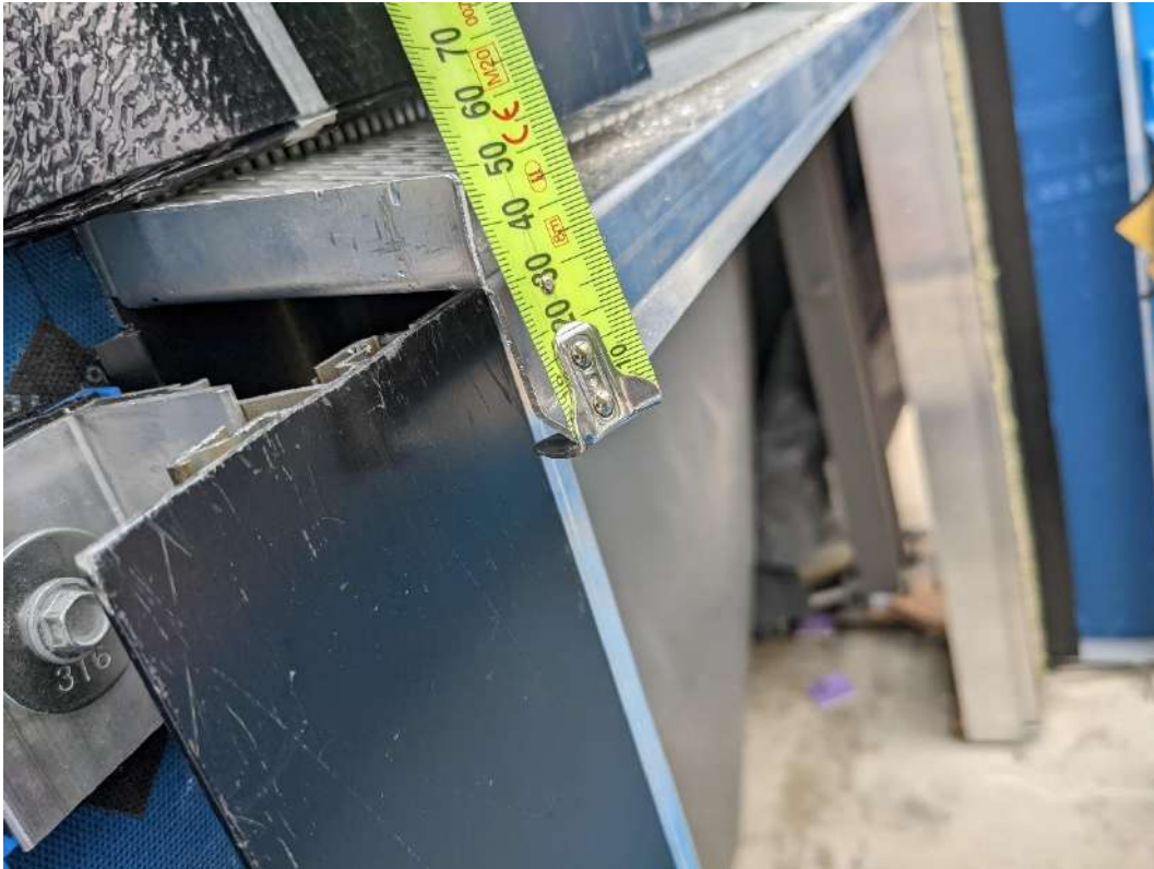
Photo 9: Combustion chamber opening flashing
