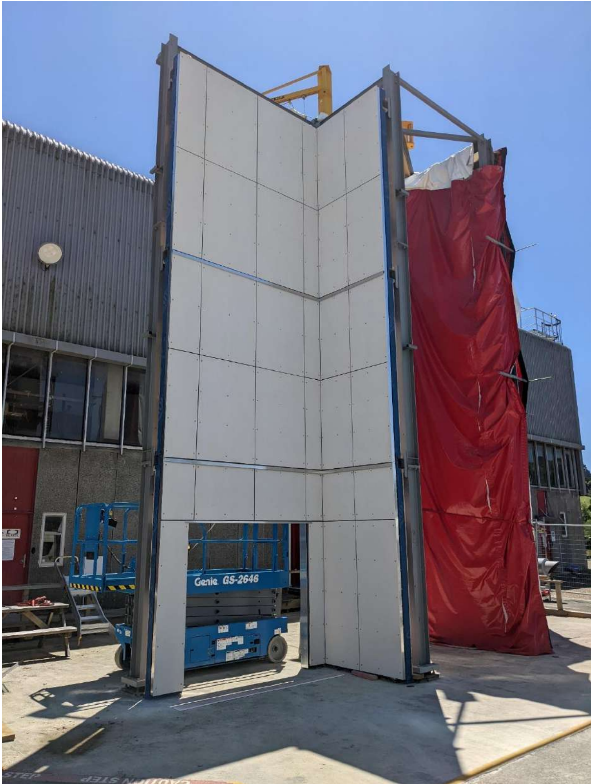
Photo 19: Completed installation (excluding parapet capping)
