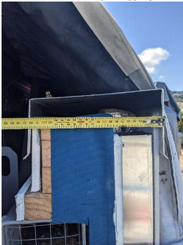
Photo 14: Parapet capping
