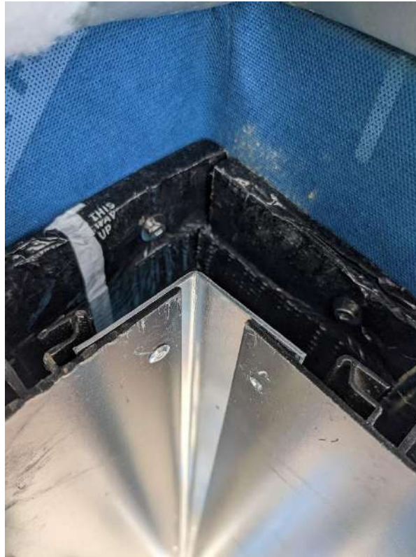
Photo 15: Internal corner panel fixing rails and horizontal fire cavity barrier
