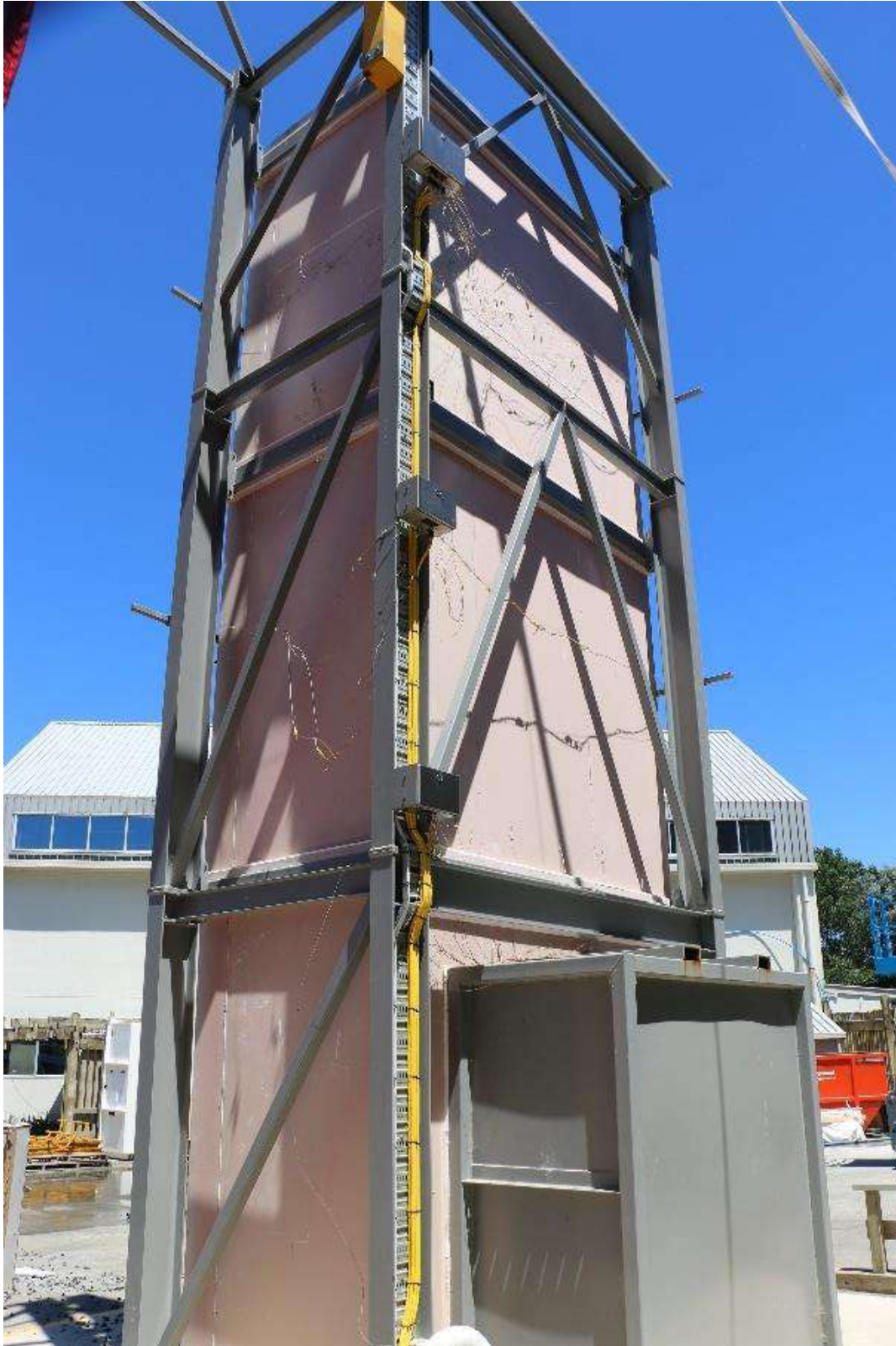
Photo 34: Post-test unexposed surface
