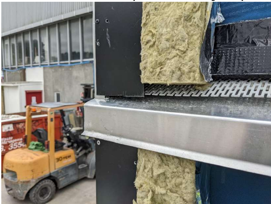
Photo 16: Vertical fire cavity barriers and drainage cavity
