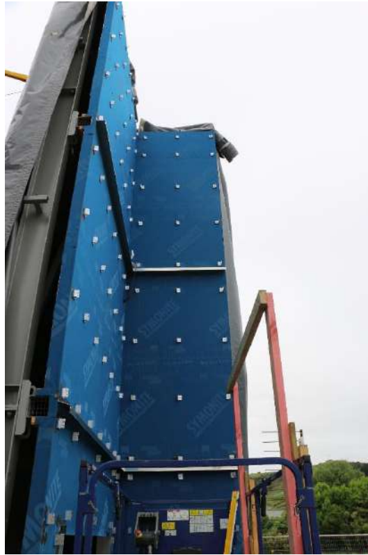
Photo 7: Waterproofing membrane, rail brackets and inter-storey drainage flashing
