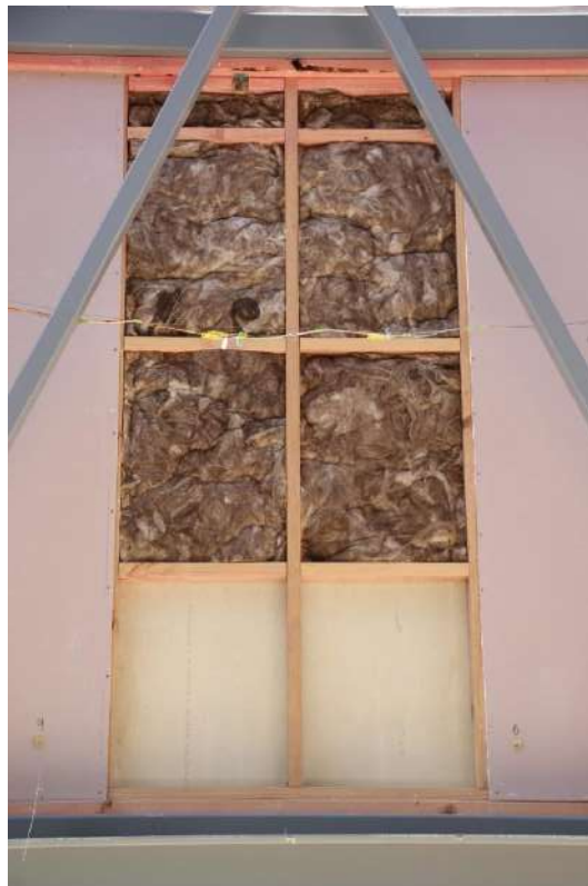
Photo 18: Insulation and internal lining
