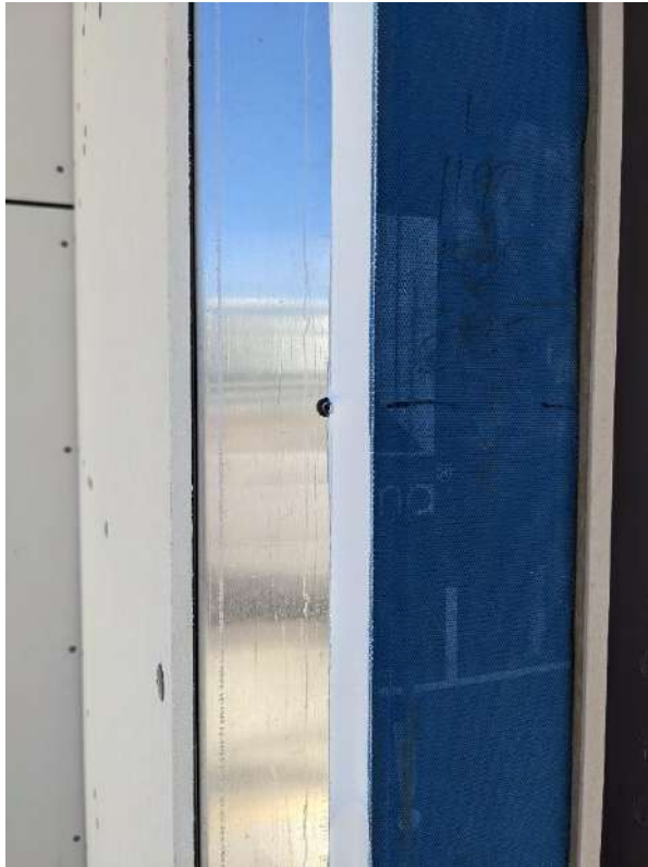
Photo 13: Wing wall edge
