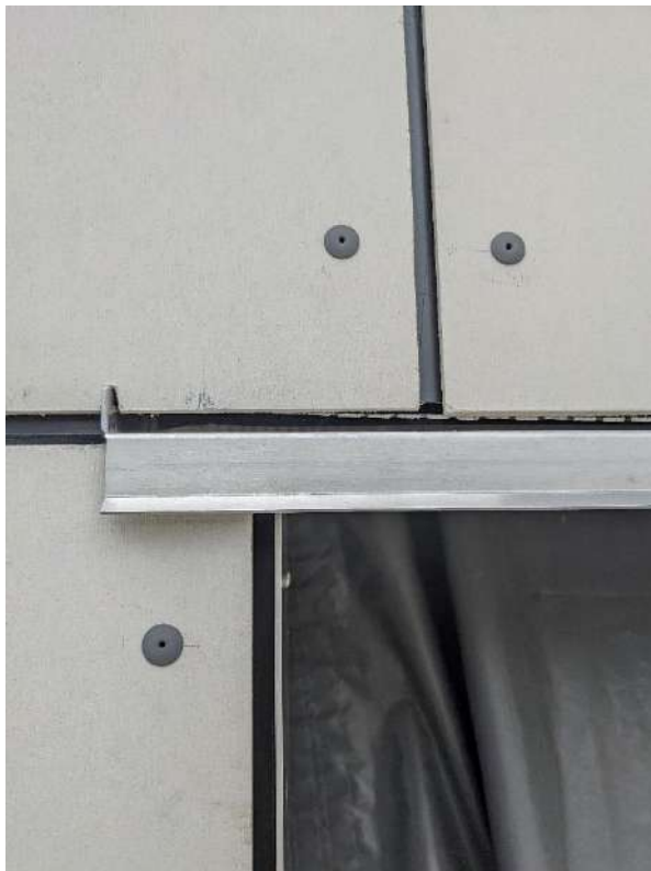
Photo 12: Combustion chamber opening; Equitone panel and aperture head flashing
