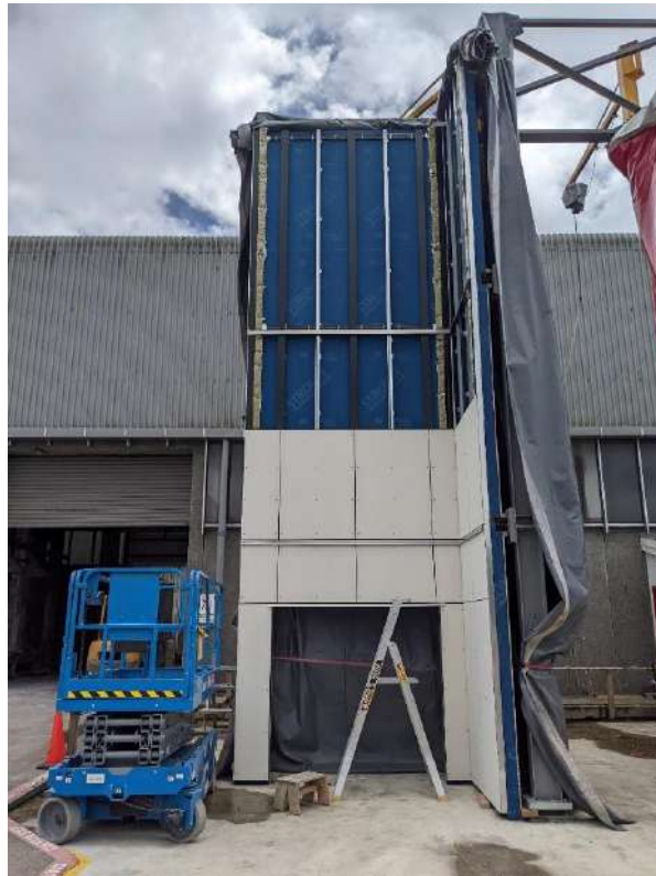
Photo 10: Equitone panels and fire cavity barriers
