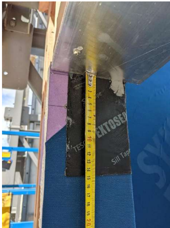
Photo 8: Combustion chamber opening sill tape and custom angle
